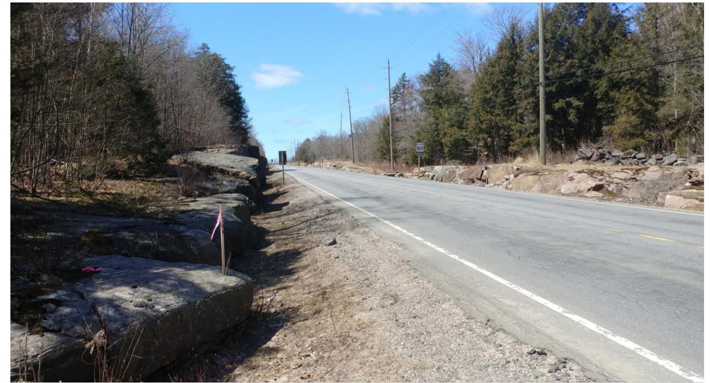
Sight lines towards the west along Highway 632 from the west site access
