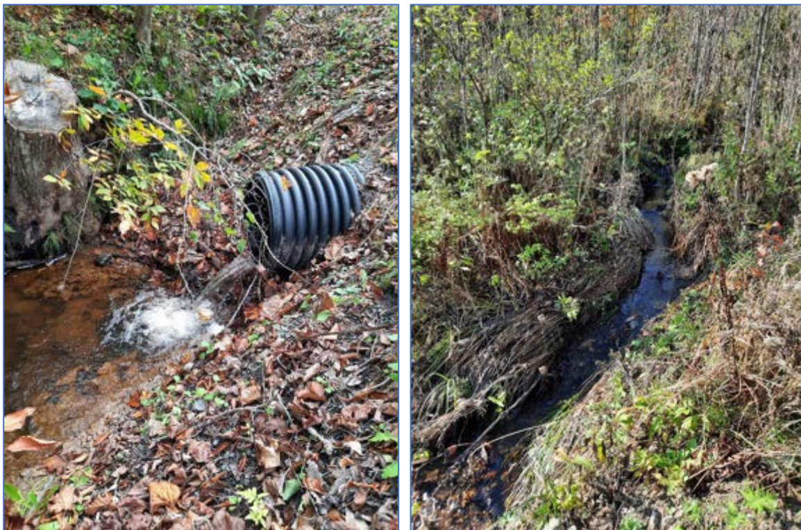
Figure 119 (left): Culvert under Maplehurst Road, downstream perch Figure 120 (right): Stream as it follows ditch line of easement road.
